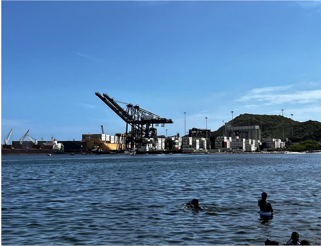
Containers terminal in Buenaventura
