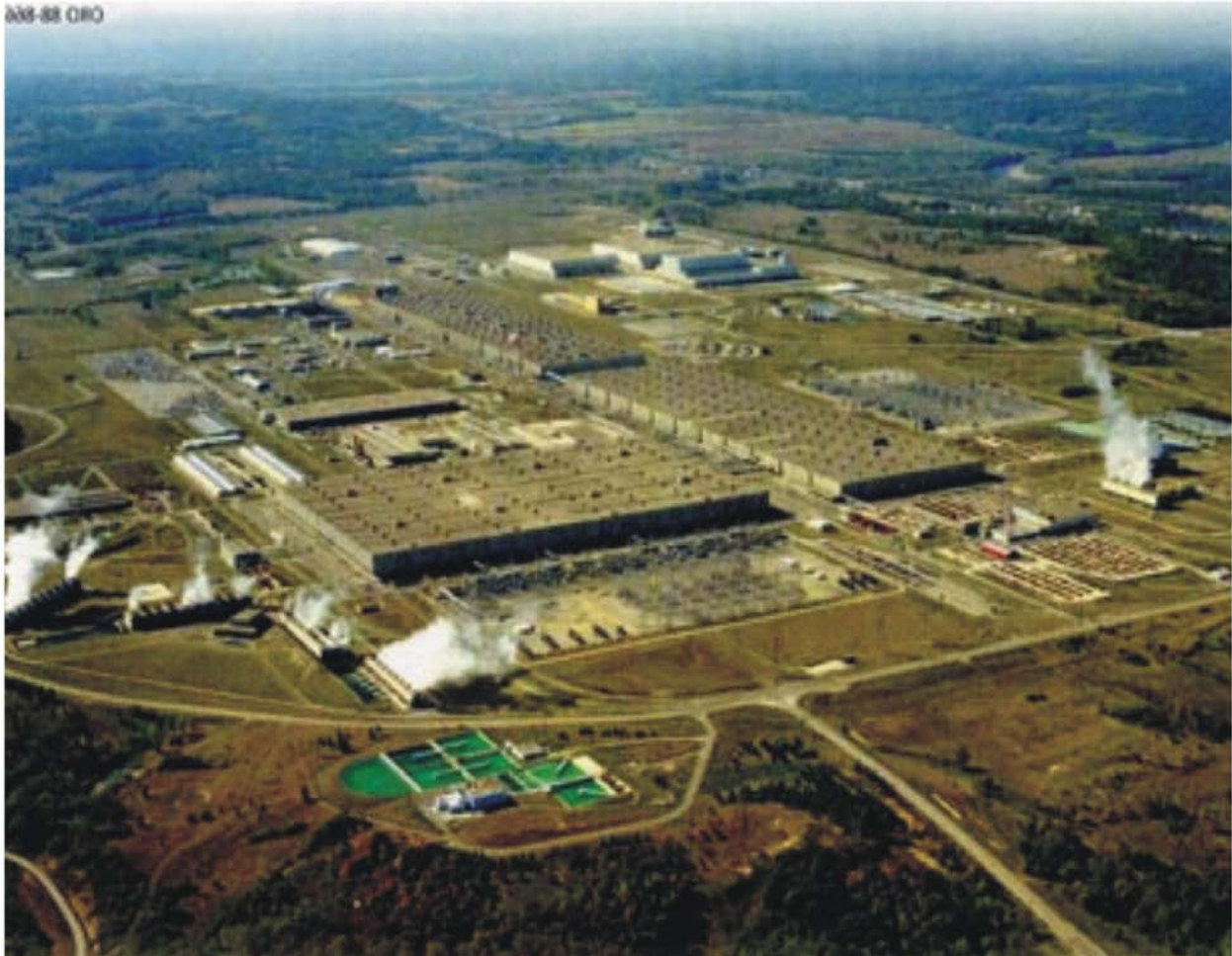
Figure 2.2-2. Photograph of PORTS from about 1988.
